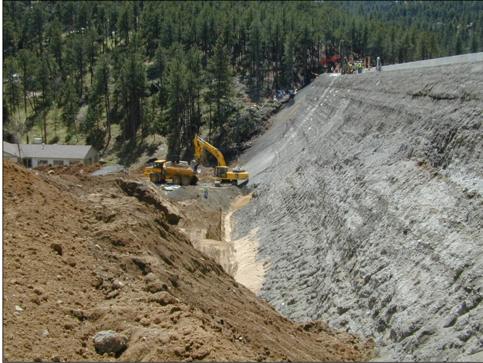
Figure 8. Unformed downstream face and installation of toe drain.
