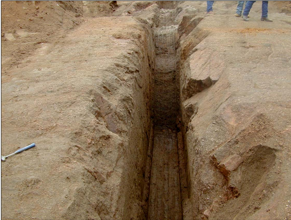
Figure 7. Foundation cutoff trench.
