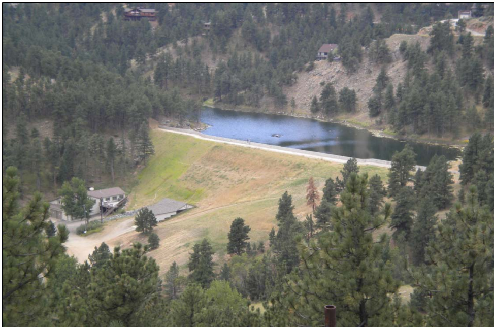
Figure 9. Completed dam with downstream soil cover.
