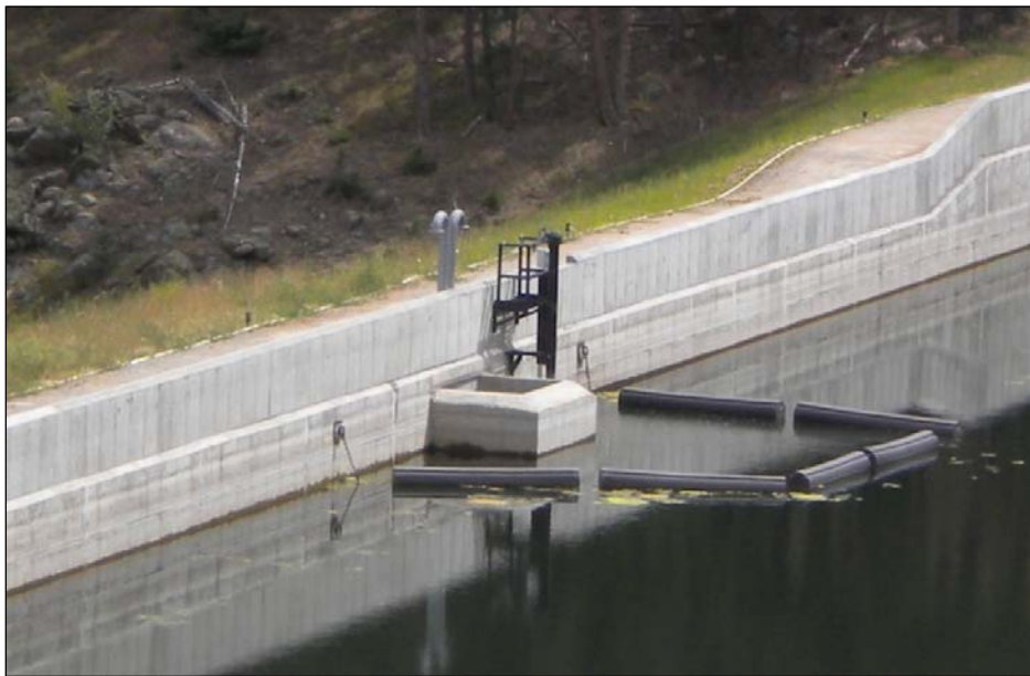
Figure 6. Service spillway on upstream face of dam.
