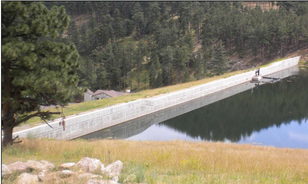
Figure 5. Upstream face of dam and emergency and service spillway.
